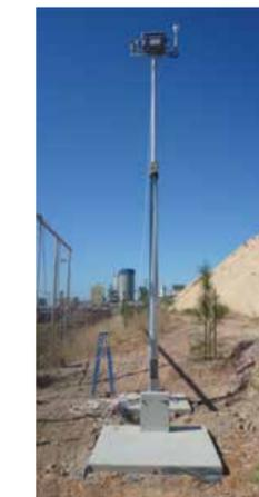
The new ambient air dust monitor located in the northeast quadrant of the Birkenhead Plant.
